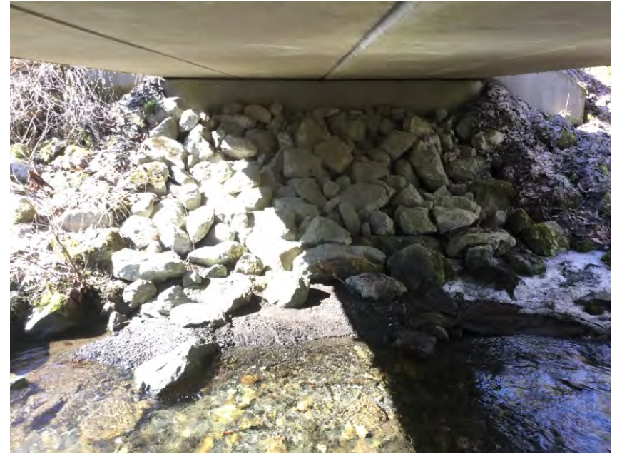
Left Bank Abutment when facing downstream
