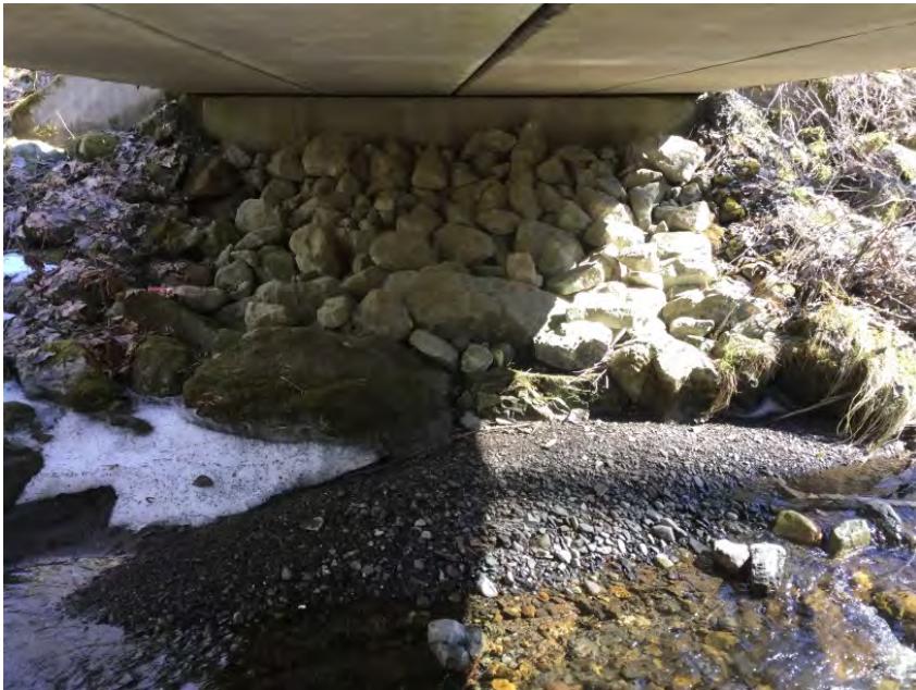
Right Bank Abutment when facing downstream
